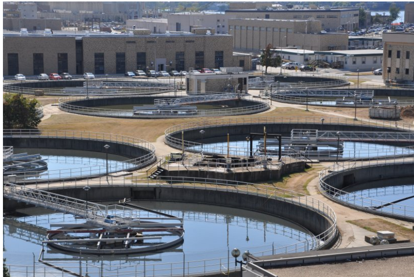
DC Water's Blue Plains Advanced Wastewater Treatment Plant. Photo courtesy of DC Water.
