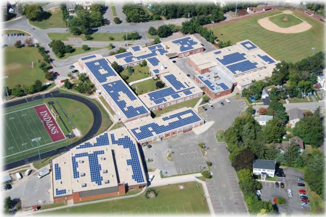
HIGH SCHOOL SOUTH
