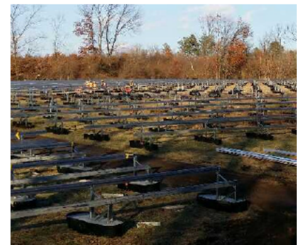
Chicopee River Solar under construction
