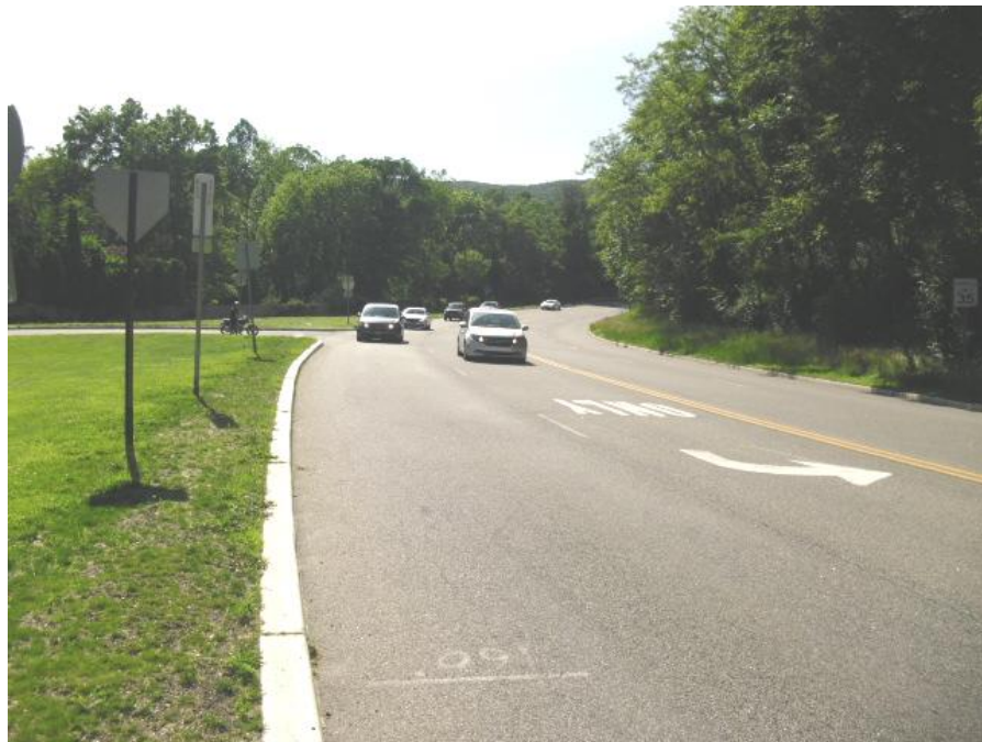
Route 202/Main Road Looking West
