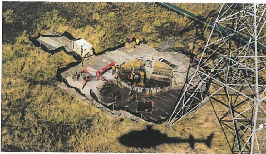
Cofferdam setup contained drill spoils from entering the wetland.
