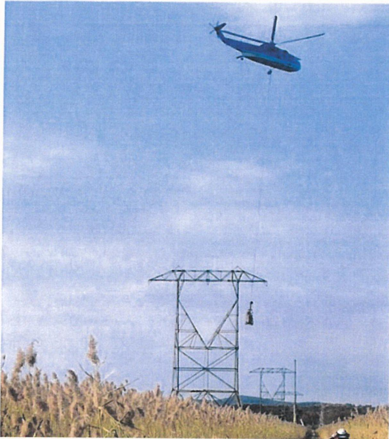
Micropile drills were transported to structure locations by helicopter.
