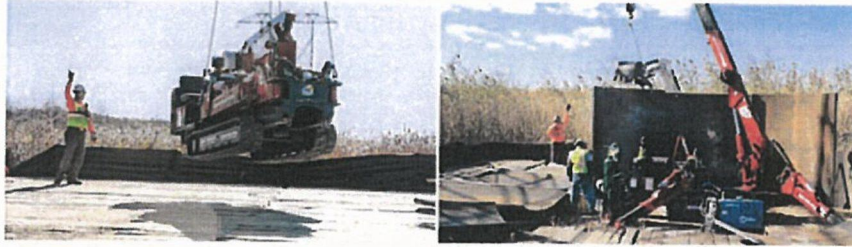
Helicopter portable cranes effectively automated heavy-lifting activities at foundation sites.
